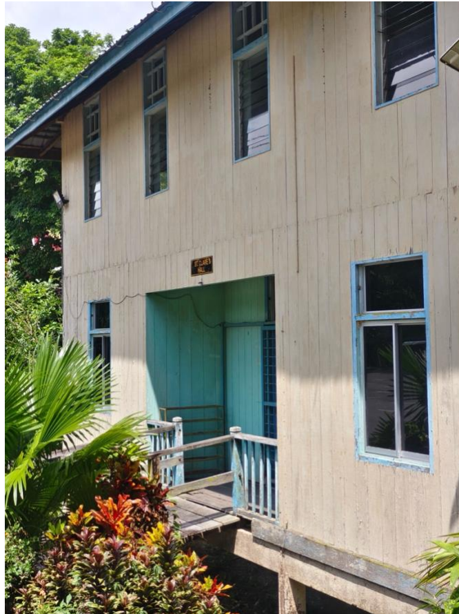
St. Clare's Hall, one of the surviving timber structures within the Kanowit mission compound. The building once served as a boarding hostel for school children attending the mission school. Photo by the author.
