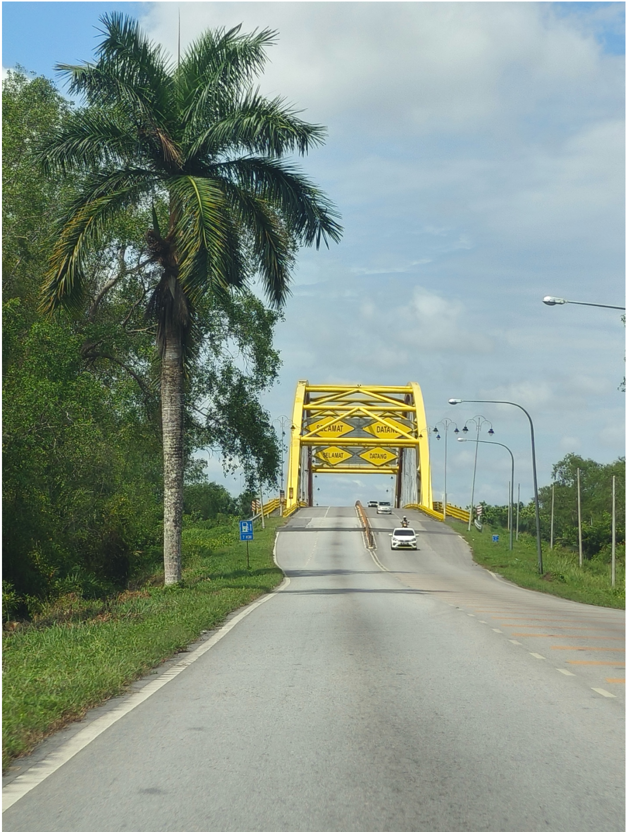
The Yellow Bridge, the gateway to Mukah Town. Photo by the author.
