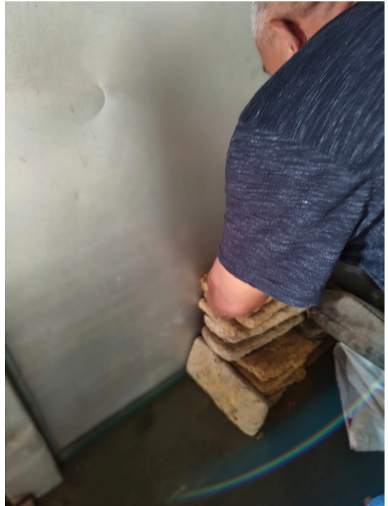
Traditional wooden moulds and clay are used to repair and reinforce the Belangan stove when cracks or damage appear from repeated heating during the roasting of sago pearls. Photo by the author.
