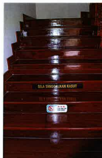
Figure 22: The wooden staircase in a heritage building portrays unique construction and is usually made of local hardwood species Source: Sanitary Board Building Conservation Project, Taiping, Perak, 2008
