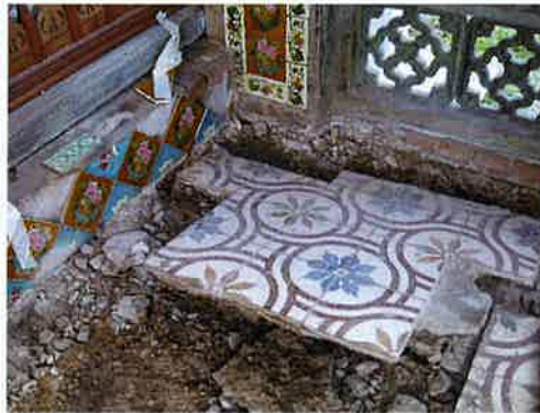
Photo 13: Conservation works on broken floor tiles Source: Penghulu Natar House Conservation Project, 2009
