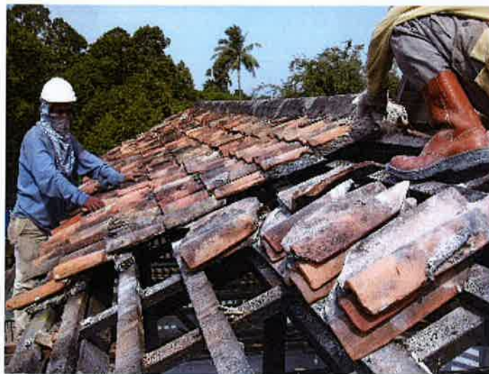
Photo 5: Disassembling the roof tiles for cleaning works Source: Penghulu Natar House Conservation Project, Merlimau, Melaka, 2009
