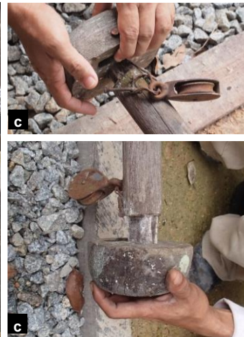
Flagpole re-assembling process. a. Upper pole was laid to the side of the lower pole. b. Fixing with timber and steel brackets. c. Upper pole was capped with a belian capping with a "built-in" pulley.
