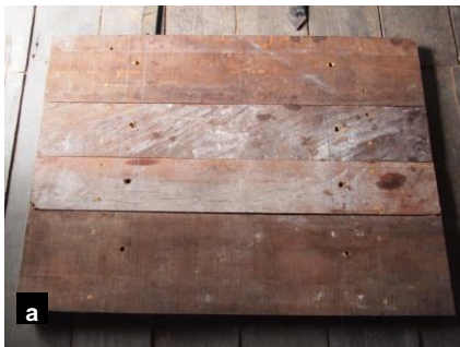
a. Pre-drilled holes on the timber door.
