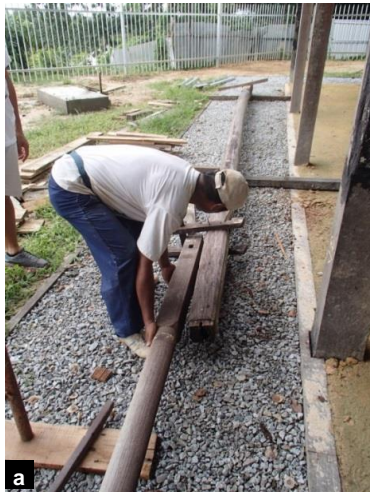
Flagpole re-assembling process. a. Upper pole was laid to the side of the lower pole. b. Fixing with timber and steel brackets. c. Upper pole was capped with a belian capping with a "built-in" pulley.
