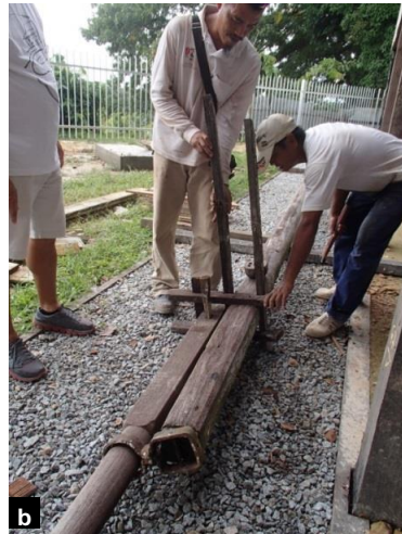
Flagpole re-assembling process. a. Upper pole was laid to the side of the lower pole. b. Fixing with timber and steel brackets. c. Upper pole was capped with a belian capping with a "built-in" pulley.
