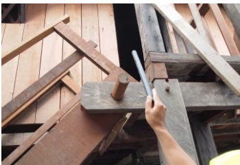
The staircase can be lifted when the 'shaft' rotates.
