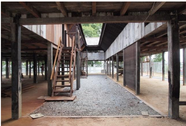
Courtyard functioning as ventilator to keep the fort cool.
