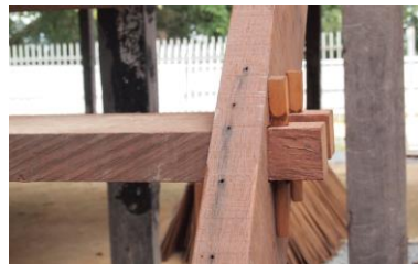
Steps are held together with wooden pegs.
