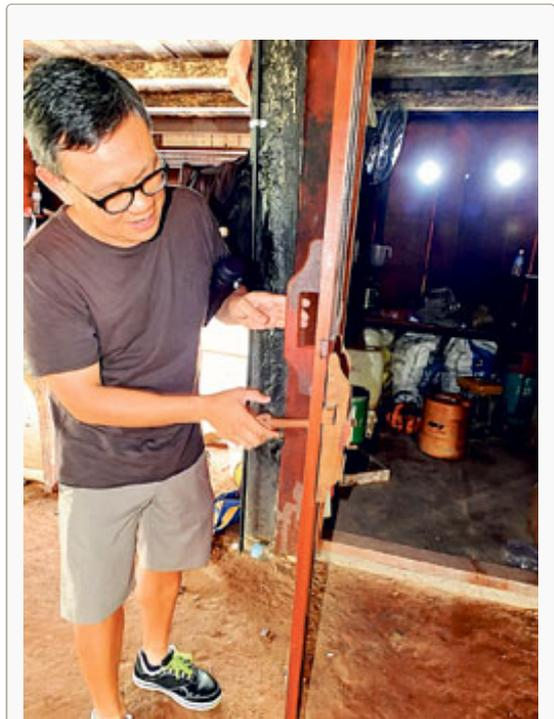
Boon shows how the locking mechanism works when the wooden key is inserted.
