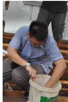
Casein melted in warm water before adding to lime wash.
