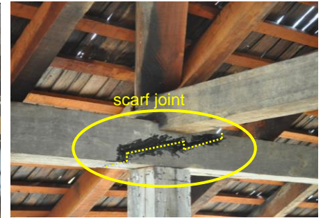
Cross-top plate and scarf joint – a traditional Chinese carpentry tradition found in old local timber construction.
