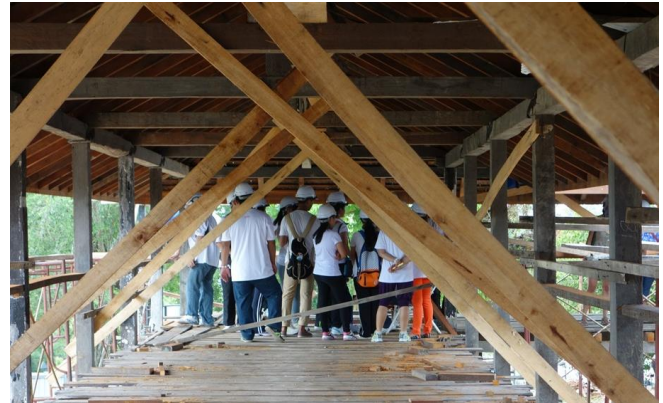
Temporary bracing for the roof framing components.
