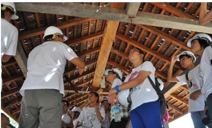
Belian shingles dismantled from the old roof were used as underlay for visual interpretation of the original roof.
