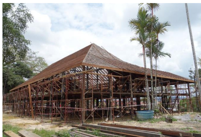
Reconstruction in progress - the roof is partially covered with belian shingles.
