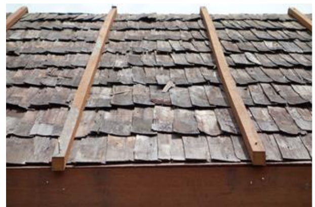
Belian shingles moved under different weather conditions. They warped when dry and levelled up when wet.
