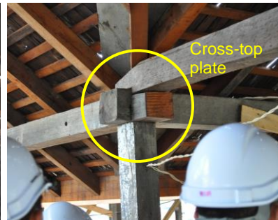
Cross-top plate and scarf joint – a traditional Chinese carpentry tradition found in old local timber construction.
