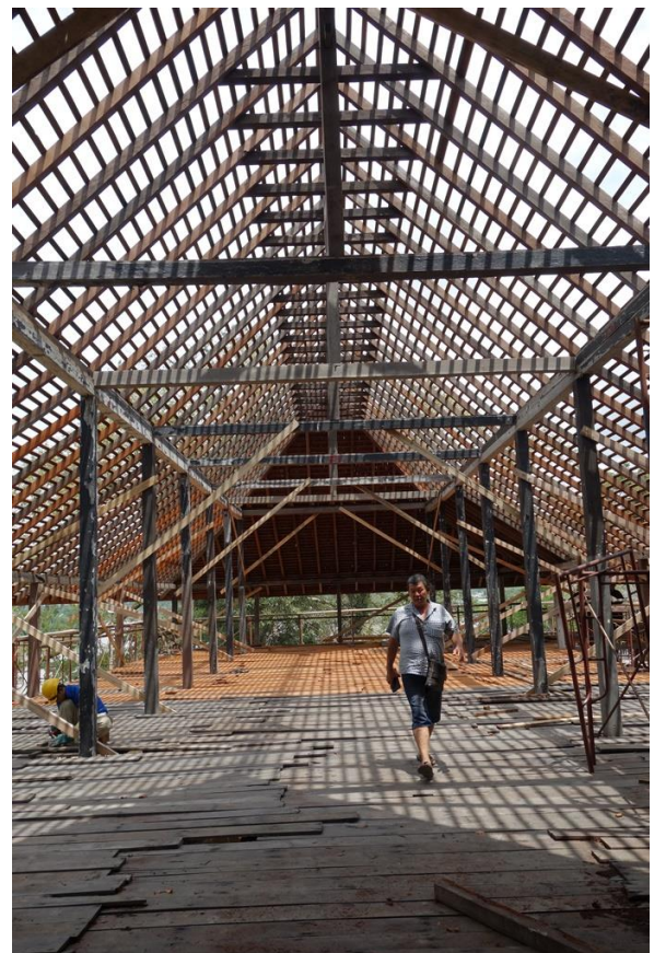
Master carpenter, Ting Nik Sing, inspecting the floor boards laid for the reconstruction of the old court room.
