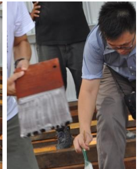
Modified lime wash applied in thin layer.
