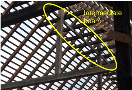
Intermediate beam - a common detail found in traditional Malay house.
