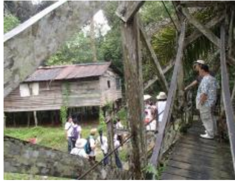
View of the kampong (village) houses on the other end of the bridge.
