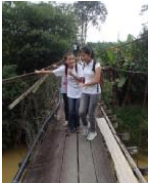
Panic-stricken while crossing the dilapidated suspension bridge.
