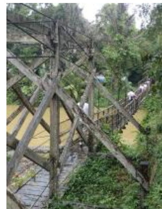
The bridge is structurally supported by (compressive) timber members and (tensile) steel cables.
