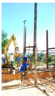
Erection of column and adjusting the verticality of the column.
