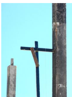
Erection of column and adjusting the verticality of the column.
