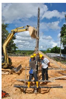
Erection of column and adjusting the verticality of the column.
