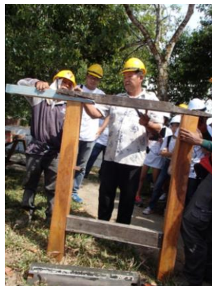
The Project's Master Carpenter Mr. Ting Nik Sing demonstrated how the timber frame of Fort Alice will be reconstructed. All the components are produced with traditional tools and techniques.
