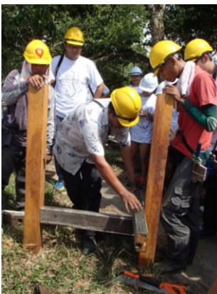
The Project's Master Carpenter Mr. Ting Nik Sing demonstrated how the timber frame of Fort Alice will be reconstructed. All the components are produced with traditional tools and techniques.
