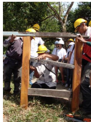
The Project's Master Carpenter Mr. Ting Nik Sing demonstrated how the timber frame of Fort Alice will be reconstructed. All the components are produced with traditional tools and techniques.
