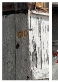
Colored codes on the timber pieces. (Yellow for main structural components, Red for secondary elements)
