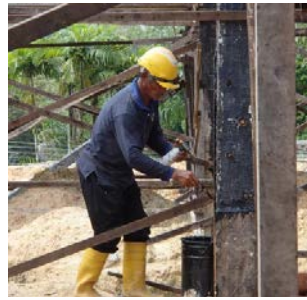
Removing excess tar with heat.
