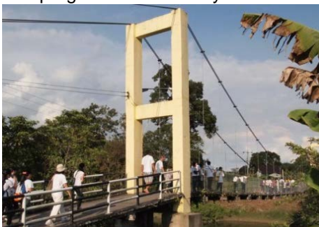
The suspension bridge in Engkilili was supported on concrete pylons.
