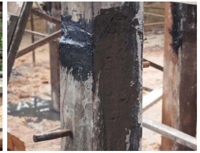
Molten tar and belian dowels at the joint.
