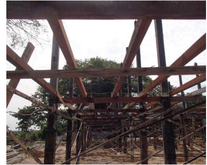
Columns, first floor bearers and joists were locked in place.
