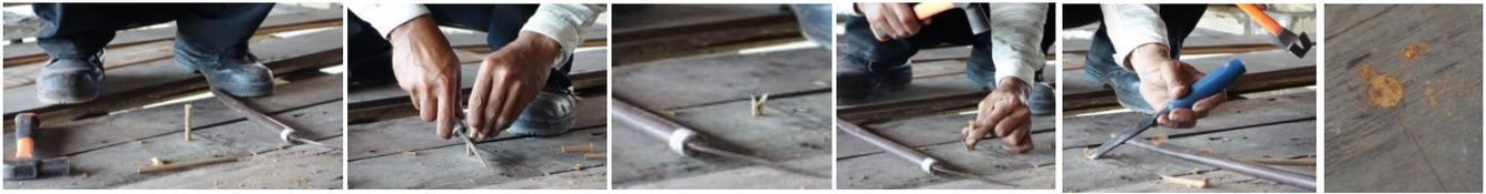
Technique of fixing floor board with a dowel (L-R) : peg the dowel into a pre-drilled hole at an angle; trim the dowel into a 'V-cut'; drive the cut-off portion into open 'V-end' until refusal; trim the expose end with chisel to flush with floor board.
