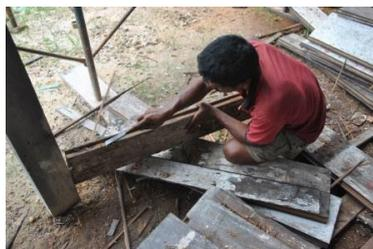
Old floor boards and wall panels were selected and processed for reuse.
