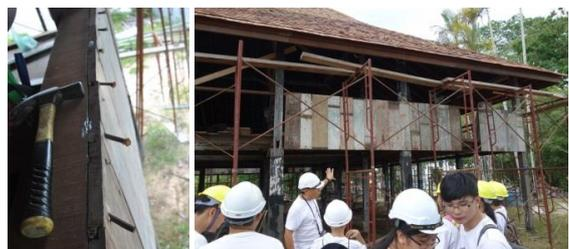
Wall panels with rebated laps are temporarily held in position with steel nails, which will be replaced with 'belian' dowels to secure the panels.
