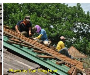
'Rockwool' and metal tray sandwiched in between belian shingles layers for insulation and water tightness.
