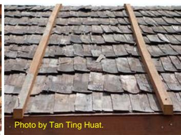
Belian shingles moved under different weather conditions. They warped when dry and levelled up when wet.
