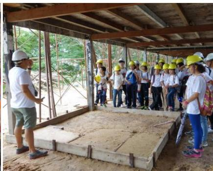
Samples of compacted clay floor prepared on site.
