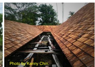
New machine-cut shingles are used for top finishing.
