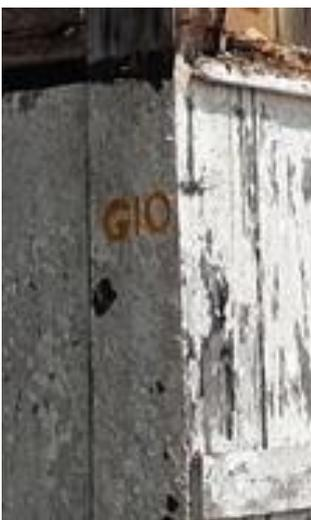
Colored codes on the timber pieces. (Yellow for main structural components, Red for secondary elements)
