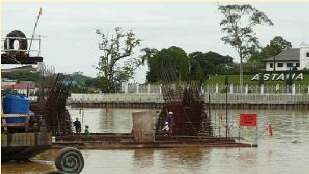
Start of construction of the 'Golden Bridge' (SHS photo-16 Nov. 2015)
